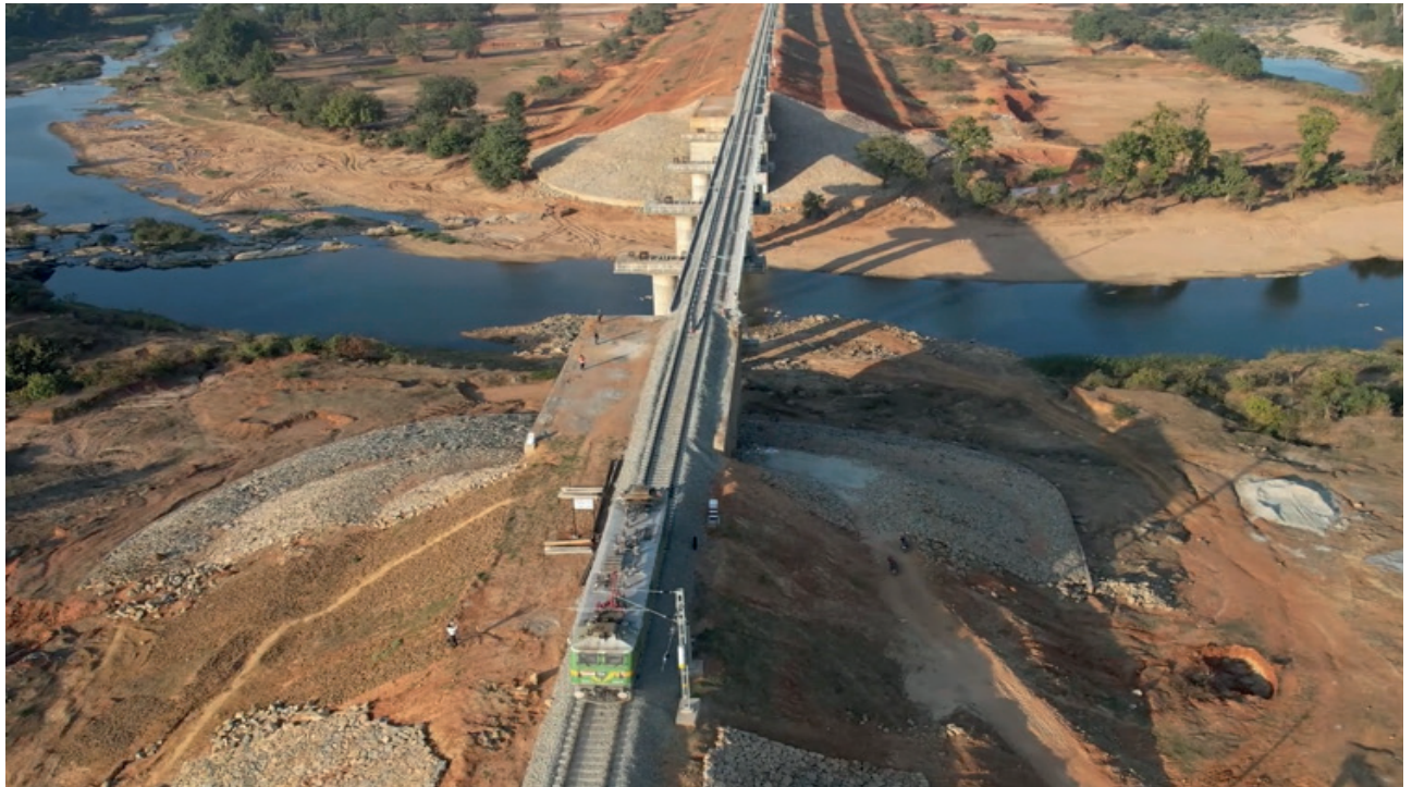
MJB-17 (CH. 10+150) BETWEEN SHAHPUR AND DUARI
