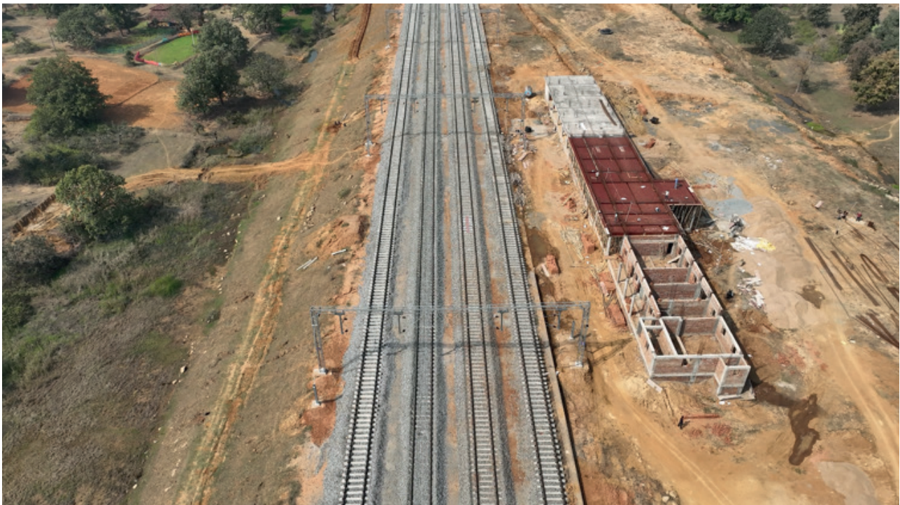
SHAHPUR YARD (CH. 6+30 KM)
