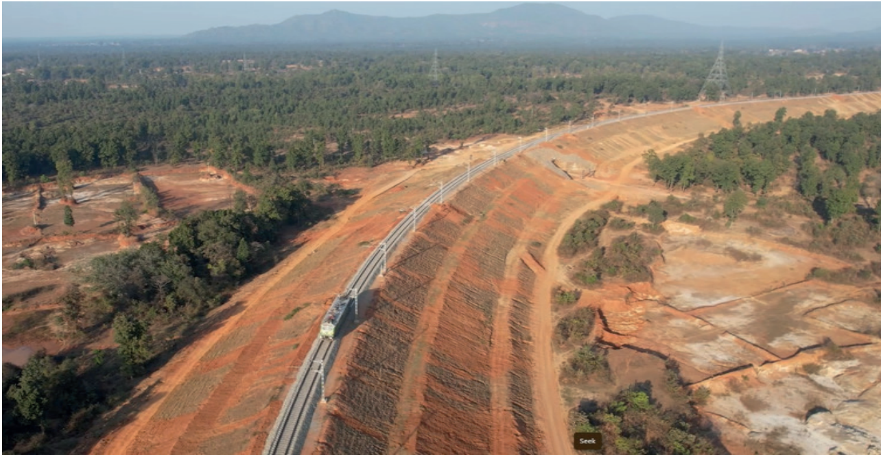
CH. 8+500 BETWEEN SHAHPUR AND DUARI
