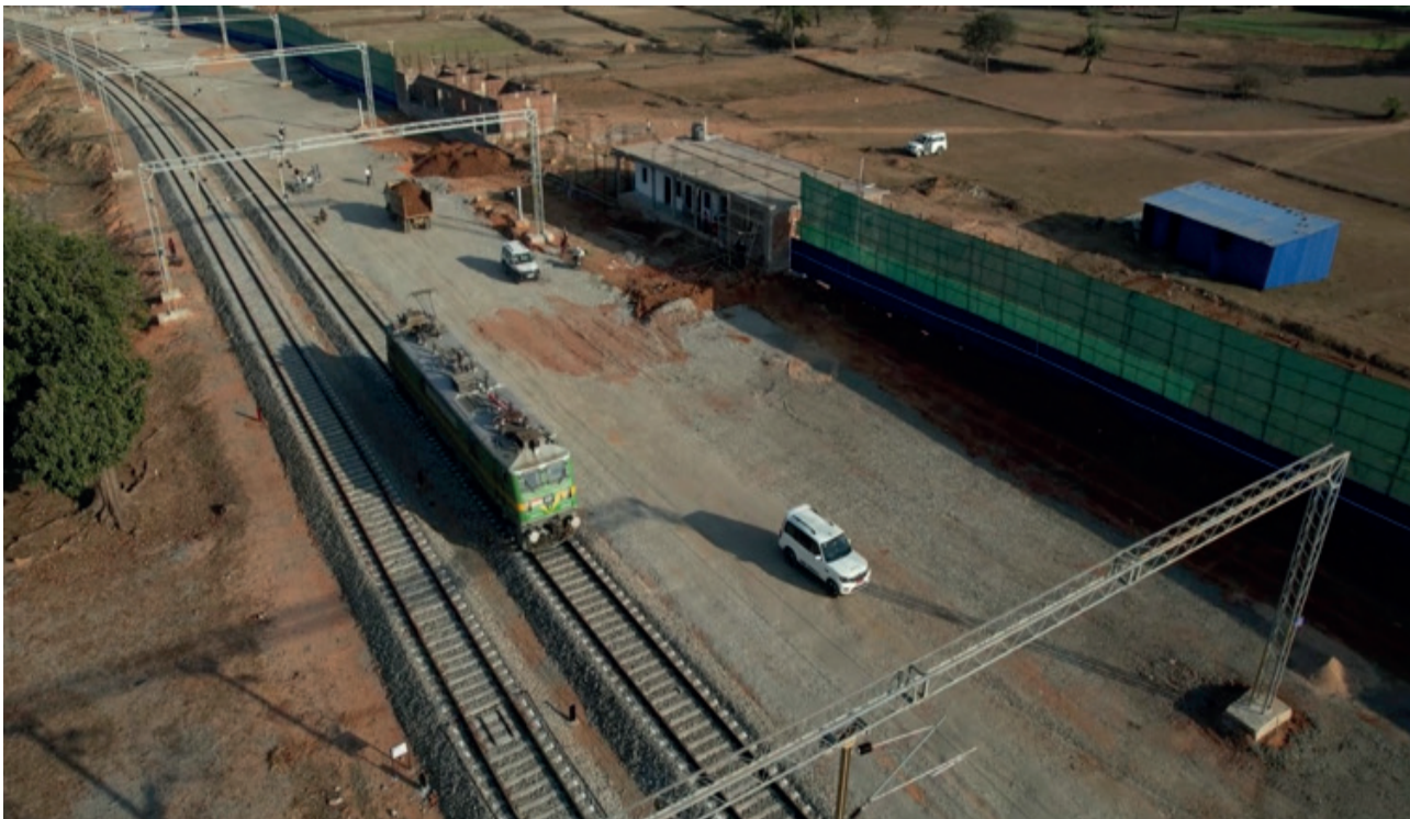
CH. 13+150 DUARI WHARF YARD
