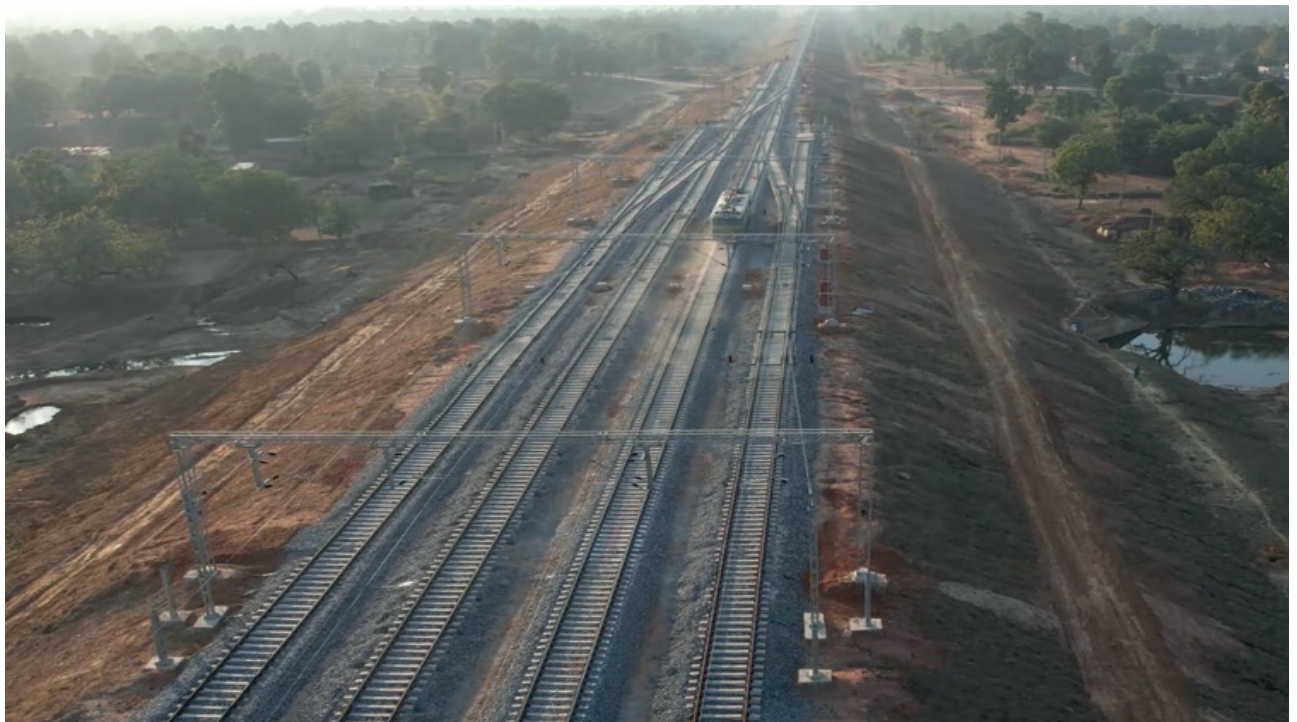
CH. 6+200 SHAHPUR YARD
