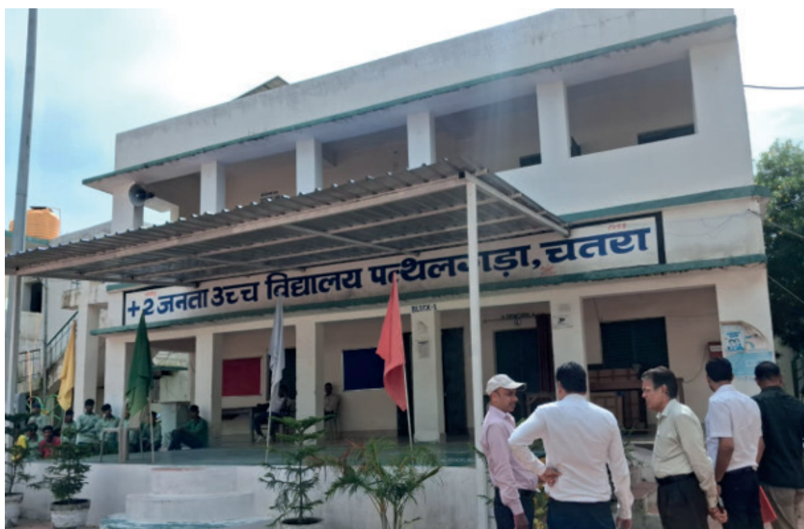
ASSEMBLY SHED INSTALLATION AT +2 JANTA HIGH SCHOOL, PATHALGADA CHATRA
