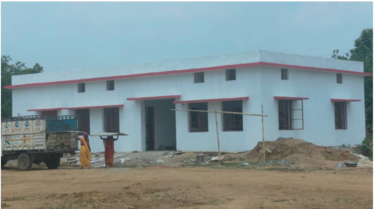
SIMARIA TSS BUILDING
